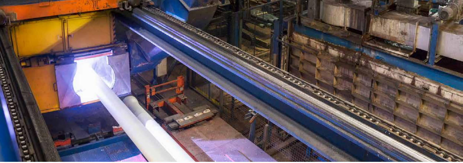
Thermal zinc spraying
